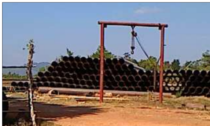
A stack of pipe segments is seen a transfer station where segments will be sent to portions of the pipeline that will be completed.
