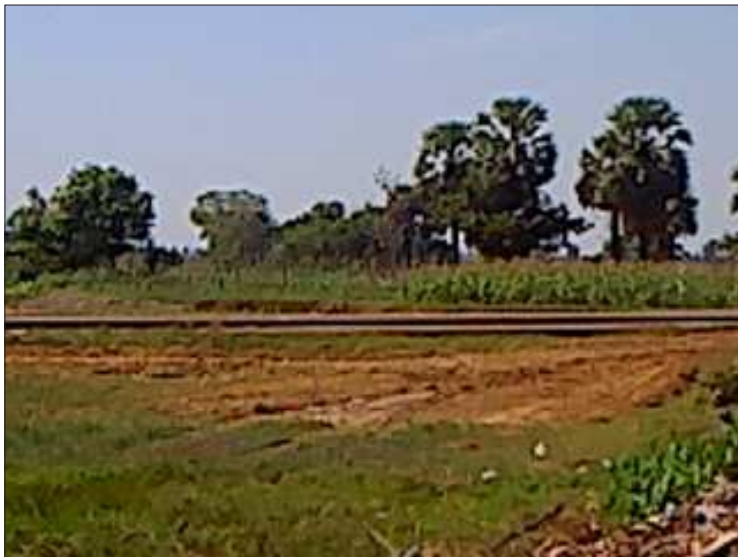
A portion of the Kanbauk to Myaing Kalay pipeline is seen outside Lamine sub-township in late February 2011.
