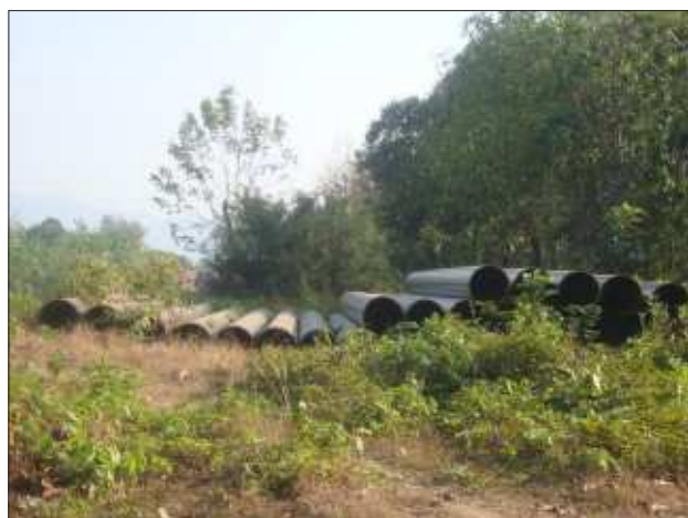
New segments of pipe for the Kanbauk to Myaing Kalay gas pipeline are seen sitting in a pile near Weakhami village, Thanbyuzayat Township.
