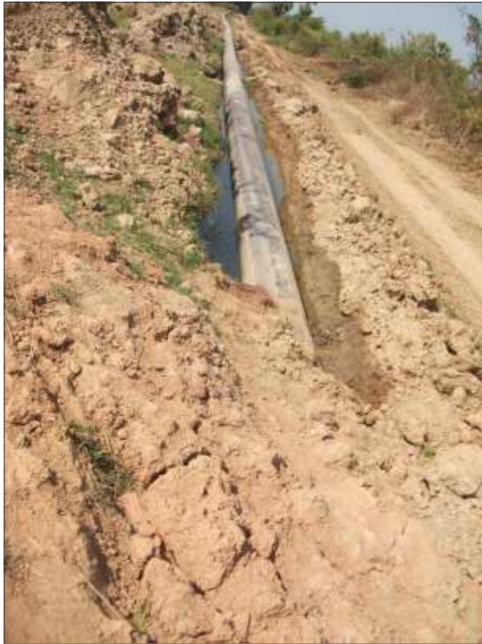
A portion of newly laid pipeline is seen recently installed, waiting to be recovered by village laborers from Lamine sub-township.
