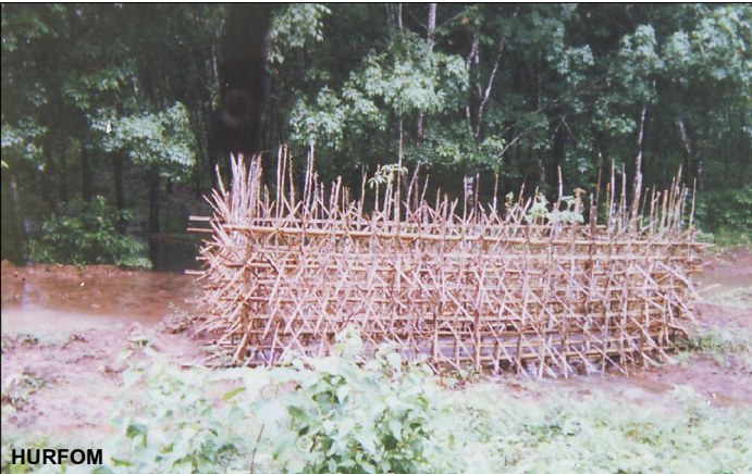
Fencing around a section of exposed pipeline in northern Ye Township
