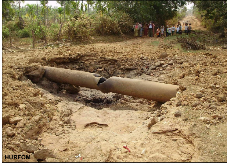
HURFOM Ruptured pipeline surrounded by a crater left by escaping gas near Lamine Town, northern Ye Township
