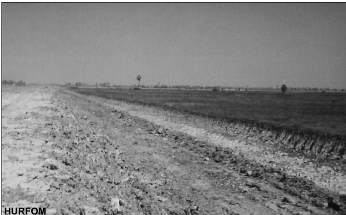
Trench dug for the pipeline during construction on the route through northern Ye Township
