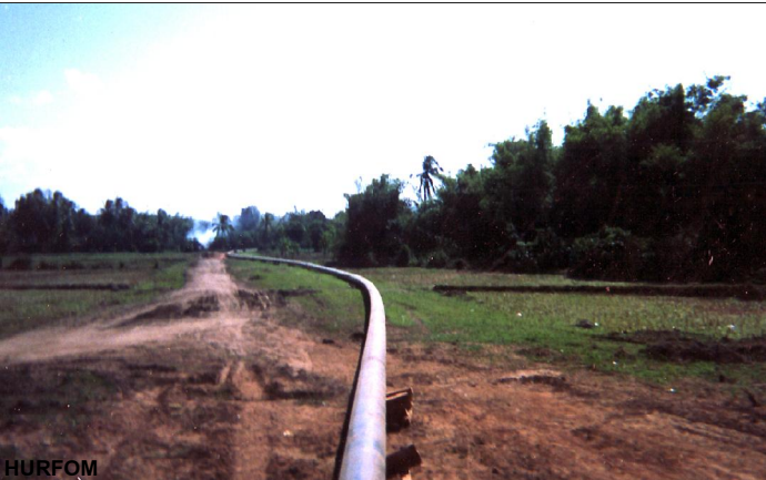
The Kanbawk to Myaing Kalay gas pipeline during construction in Ye Township
