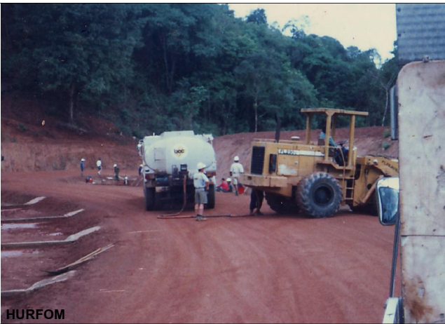
Construction of the Total Pipeline Center near Kanbauk, Tenasserim Division
